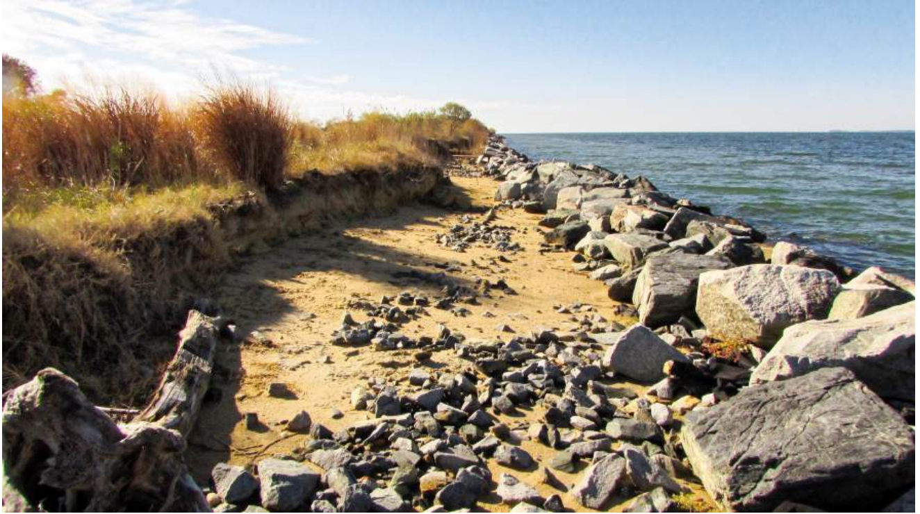
Behind the riprap
