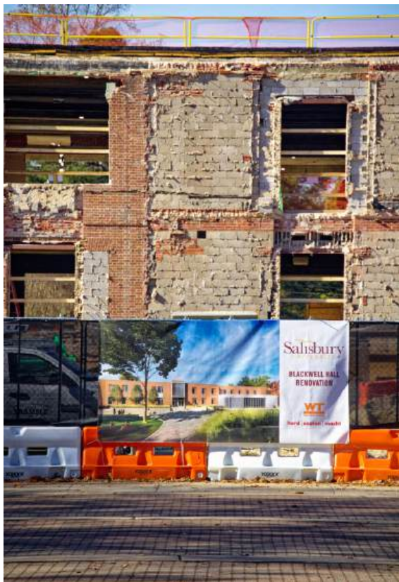
Blackwell Hall renovation Photo: Jay Goodman
